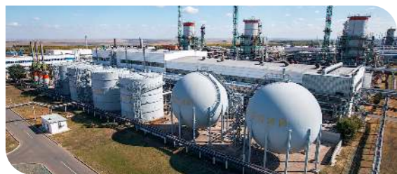
GAZPROM DOBYCHA ORENBURG HELIUM PLANT (RESTORATION AFTER A TECHNOLOGICAL ACCIDENT) Commissioned in 2009
