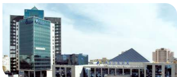
GAZPROM DOBYCHA ORENBURG GAZPROM-CITY SOCIAL AND BUSINESS COMPLEX Commissioned in 2011
