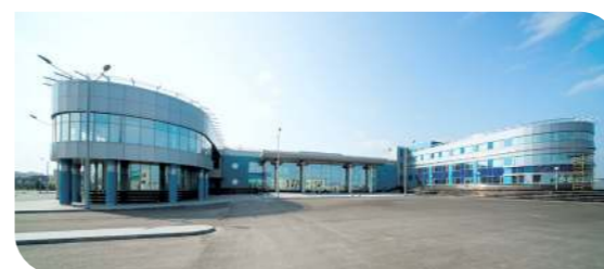
MULTIFUNCTIONAL STATION, NEW URENGOI Commissioned in 2015
