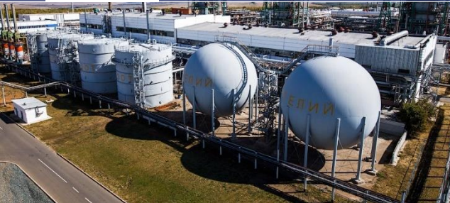
Reconstruction of the Orenburg helium plant
